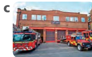
at a fire station
